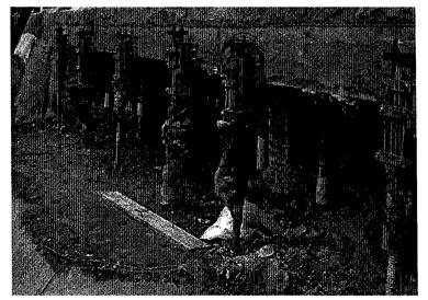
advantages over traditional pilings, such as the speed of installation, little noise and minimal vibration that may cause damage to the surrounding area.
